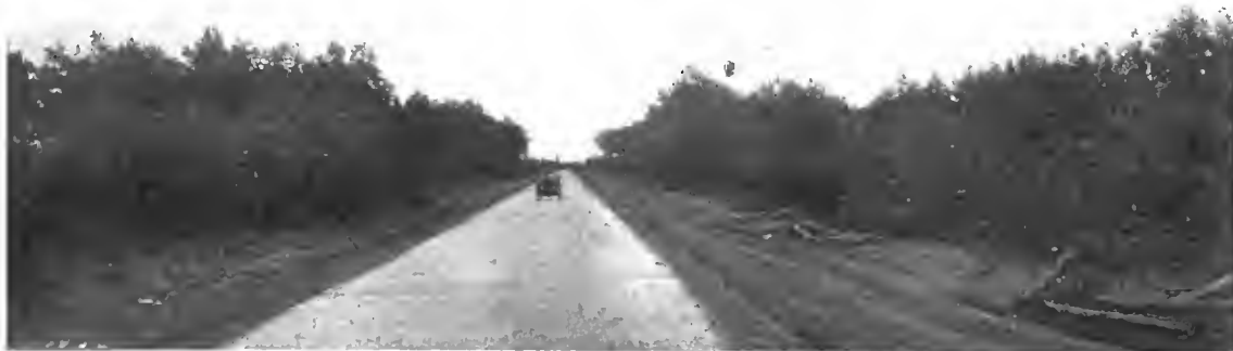
One of the Nearly Completed Stretches of the Long Island Motor Parkway, That Will be Used in Vanderbilt Cup Race.
